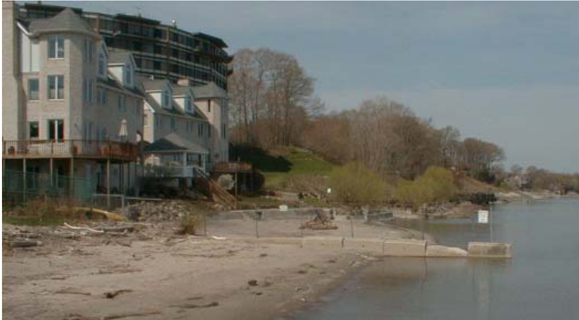
Photo 1 May 5, 2005 at a location in Rocky River.
