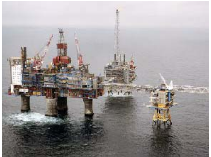
The Sleipner CCS project in Norway has been injecting CO 2 underground since 1996, and sequesters about one million metric tons of CO 2 each year.
