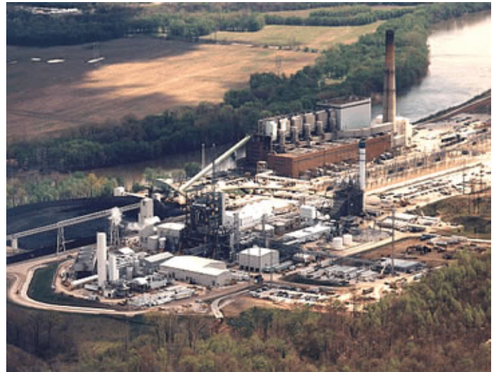
IGCC promotes the adoption of the coal power production methods that produce the most minimal environmental impact. (IGCC plant at Wabash, IN pictured above)
